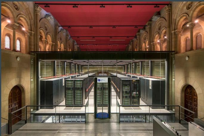
Barcelona Supercomputing center
